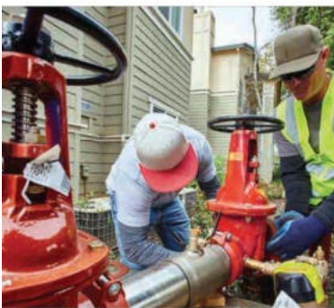
LF009 Reduced Pressure Zone Assembly
