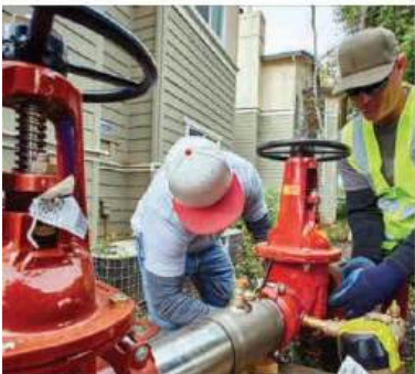
LF009 Reduced Pressure Zone Assembly
