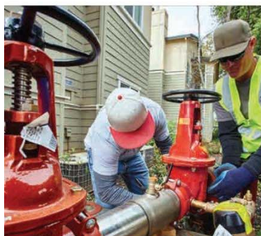
LF009 Reduced Pressure Zone Assembly
