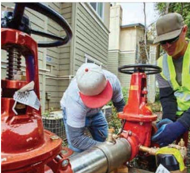
LF009 Reduced Pressure Zone Assembly
